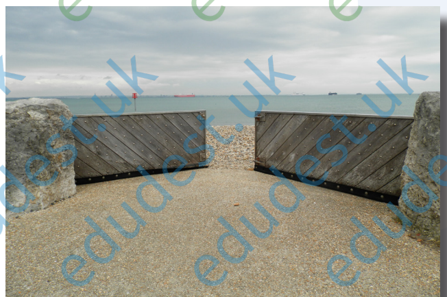
Limestone gate portals and heavy marine hardwood gates with stainless steel frames, Seaview Duver
