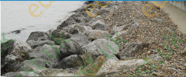
Curved sea wall, rock revetment and rock groyne at Seaview
