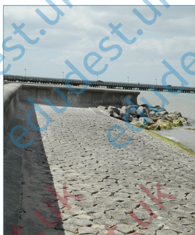
Curved sea wall and rock armour at Ryde
